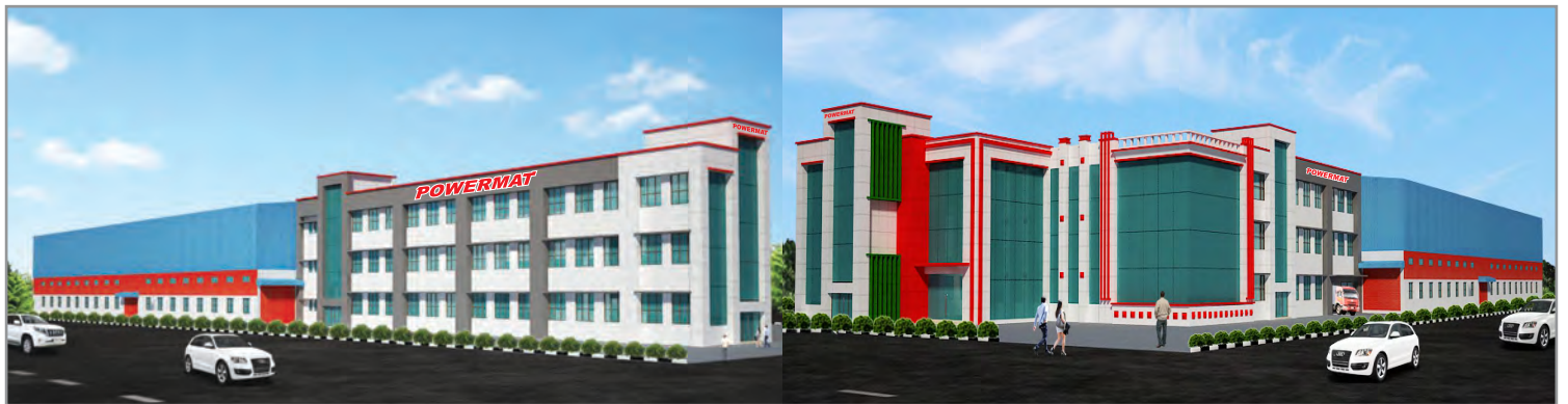
EXISTING PLANT IN BAHADURGARH (HARYANA)
